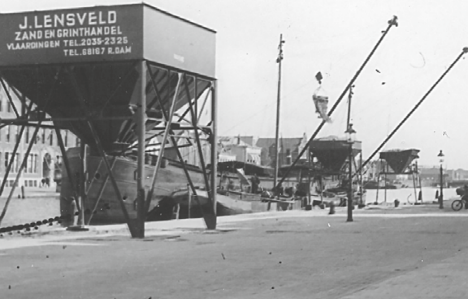
Sandbarge for the Lensveld sand hoppers.
