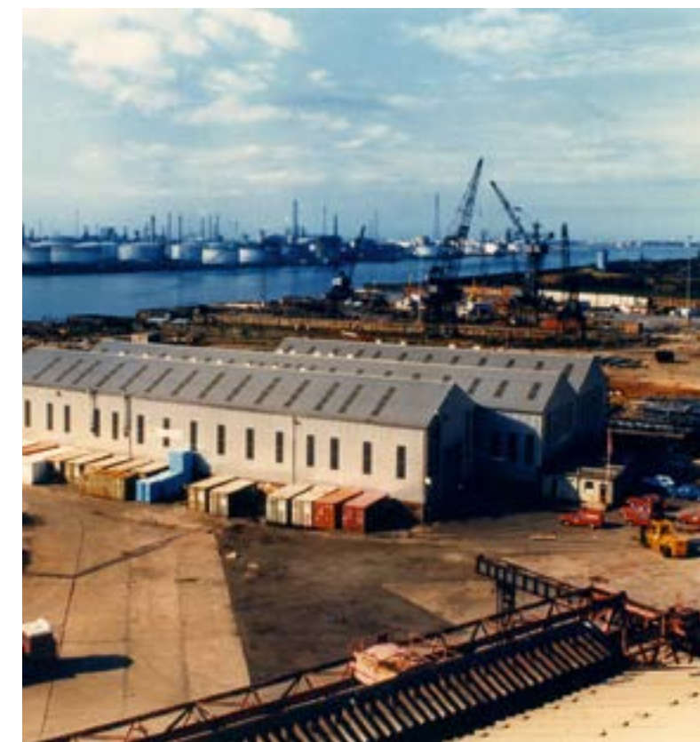
Teesport warehouse and office in Middlesbrough.
