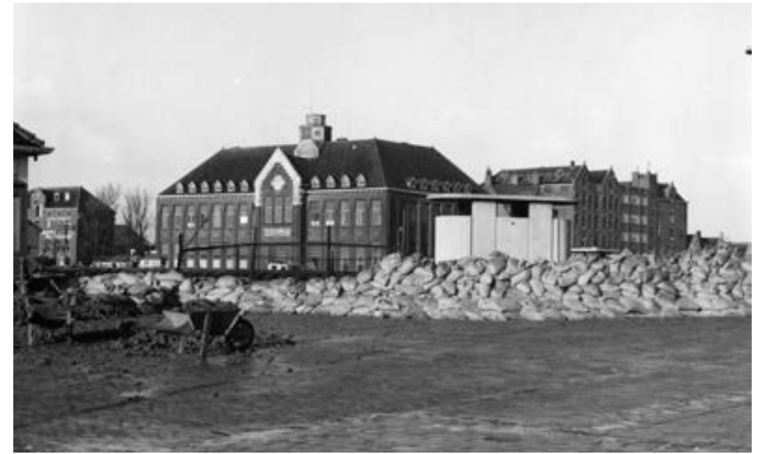
Putting up sandbags in Vlaardingen against the rising water, February 1953. Vlaardingen City Archives collection.
