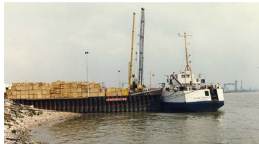
Loading and unloading at the Waterleidingstraat site.
