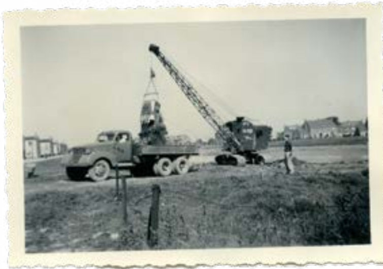
Unloading sand from a GMC CCKW with one of Lensveld's Ruston Bucyrus draglines.
