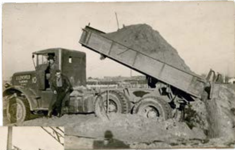
Dumping sand in a MACK NM 6-tonne truck.
