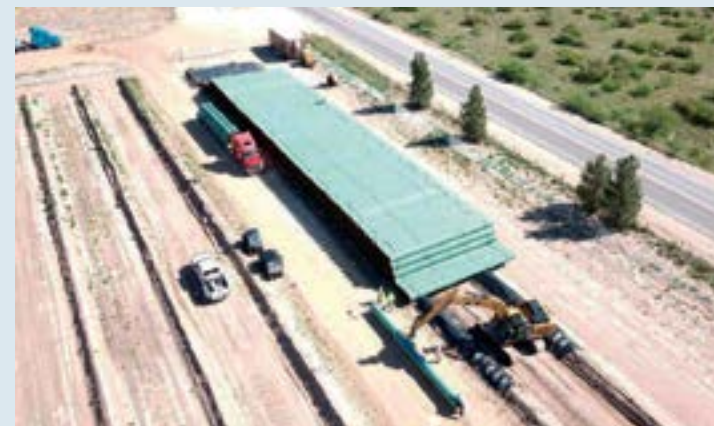
The unloading of pipes with a shovel. Kermit, Texas, 2016.
